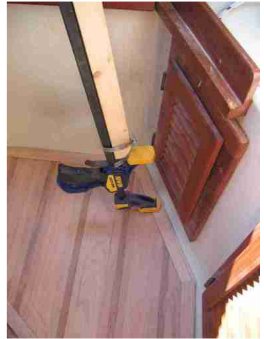
Photo 6 Close up of Cap Plank and Irwin Clamp
